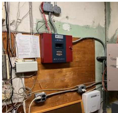
FIRELITE ALARM INC. FIRE ALARM CONTROL PANEL MODEL MS 5024
