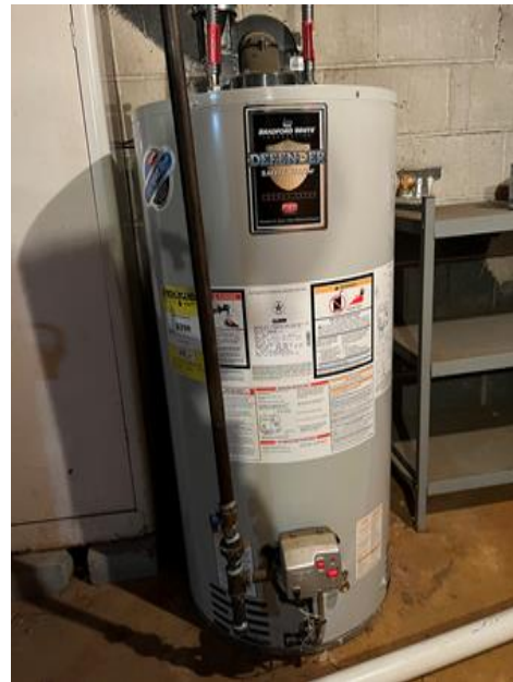
BRADFORD WHITE 40,000 BTU NATURAL GAS-FIRED BASEMENT WATER HEATER – PURCHASED 2014
