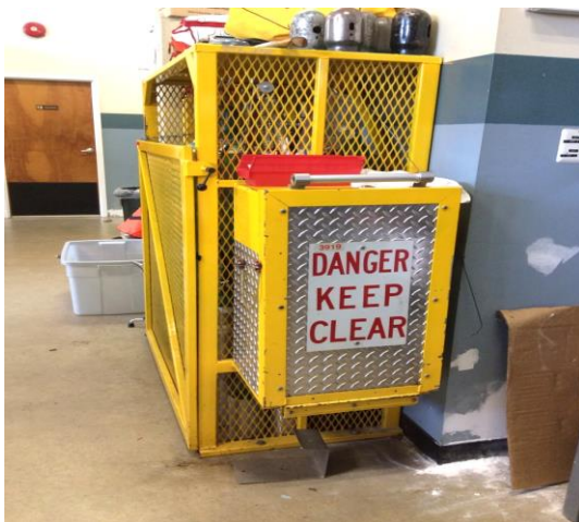
EMERGENCY SQUAD OXYGEN FILL & STORAGE CAGE
