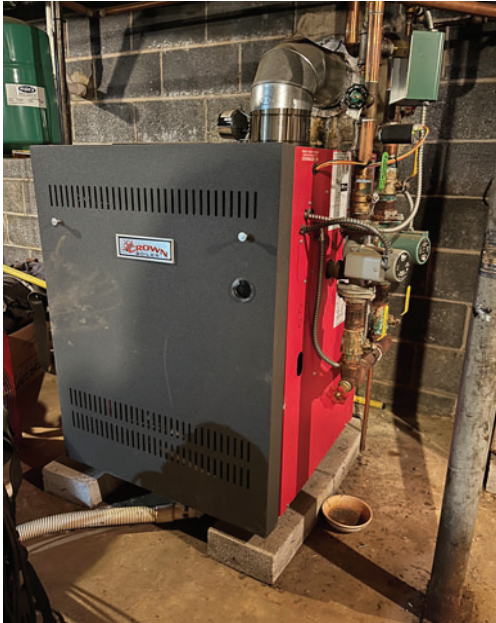
BASEMENT CROWN 245,000 BTU NATURAL GAS-FIRED BOILER LAST DATED INSPECTION 07-30-20 -- PURCHASED 2014
