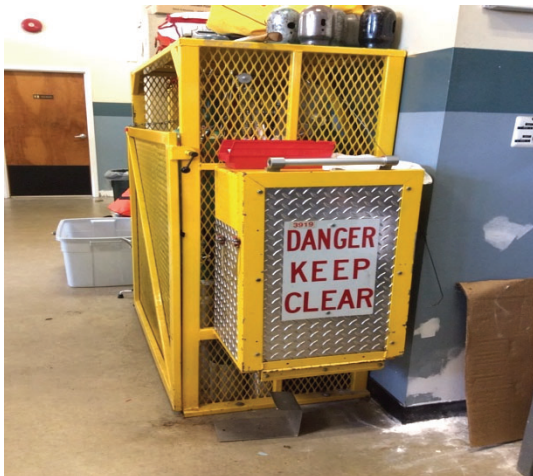
EMERGENCY SQUAD OXYGEN FILL & STORAGE CAGE
